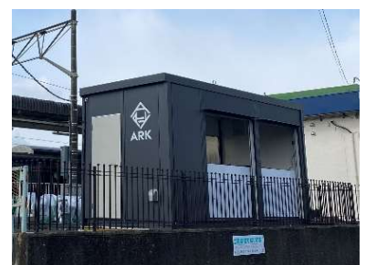
(浪江駅陸上養殖設備)
