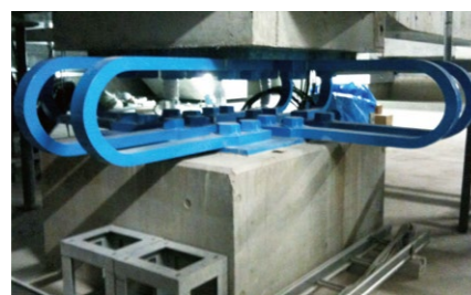
U型鋼材ダンパー U-shaped steel dampers
